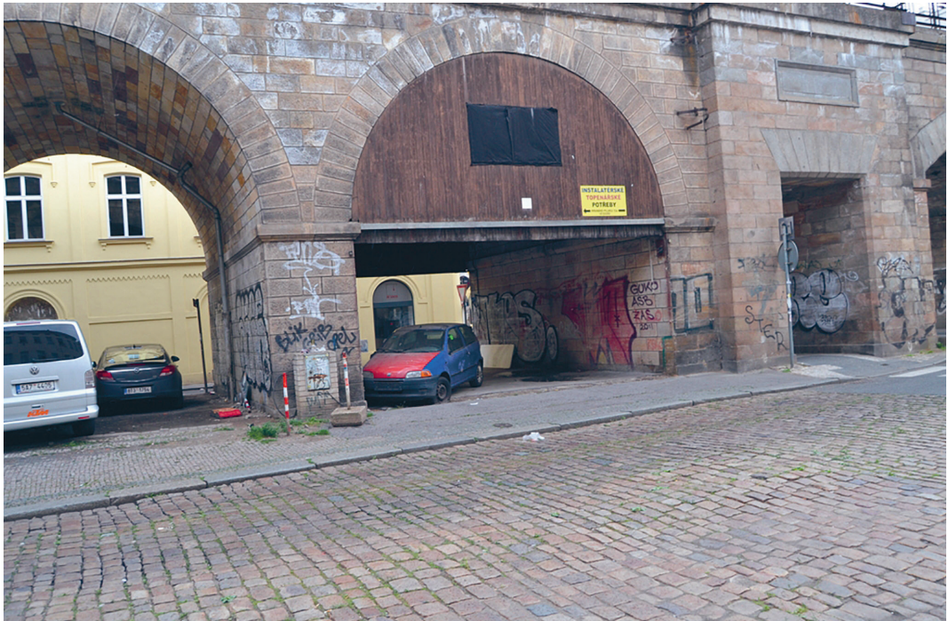
ATMOSPHERE OF THE VIADUCT BEFORE CCEA INTERVENTIONS
